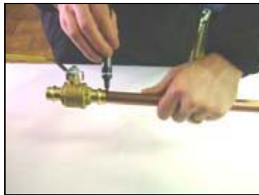
E. Using a marker, draw a line on the tubing where it enters the valve (marking the full insertion depth).
