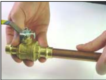
D. Turning slightly, slide press valve on to tubing to the fitting stop. Note: end of tubing must be fully inserted.
