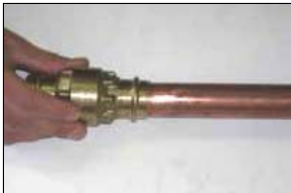
D. Turning slightly, slide press valve on to tubing to the fitting stop. Note: end of tubing must be fully inserted.
