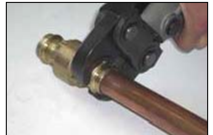
I. After pressing, release the jaws and remove the tool. Do not attempt to adjust the valve on the pipe after pressing.
