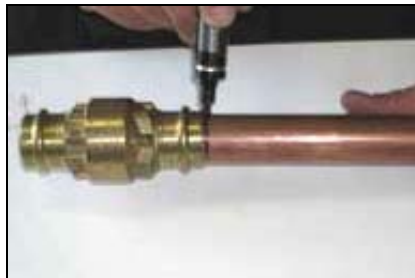
E. Using a marker, draw a line on the tubing where it enters the valve (marking the full insertion depth). Make sure that the arrow on the body is in the direction of flow.
