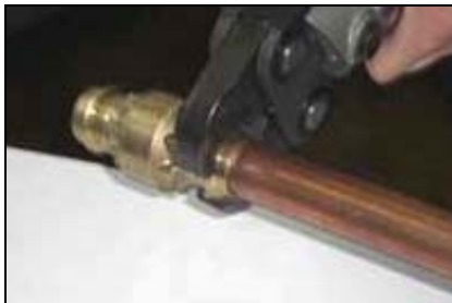
H. Start the pressing process and hold the trigger until the jaw has engaged the fitting.
