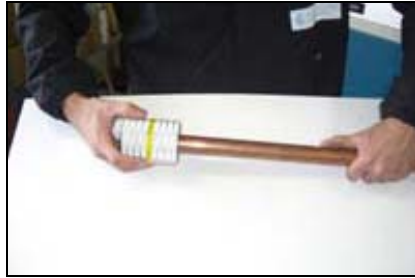
B. De-burr tubing on the inside and outside to prevent cutting of the valve's o-ring seals.
